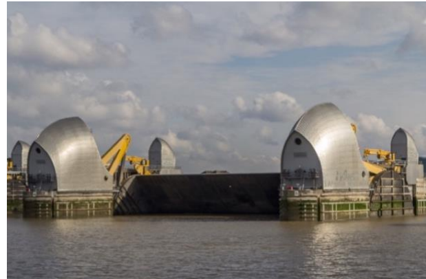
Steel gate rotated up
