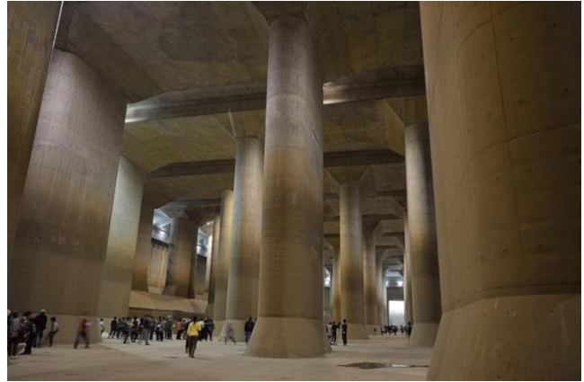
Metropolitan Area Outer Underground Discharge Channel, Japan
